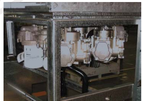
Encore with T19976-G5 Flex Fuel Meter
