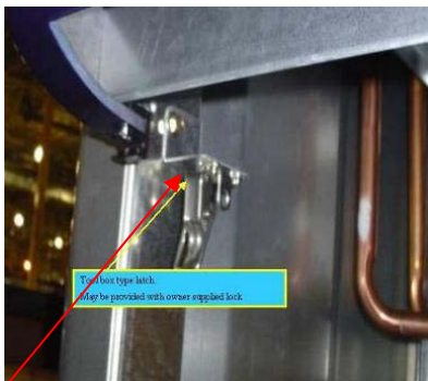
Nxx Series Tool Box Type Latch (may be provided with owner supplied lock)
